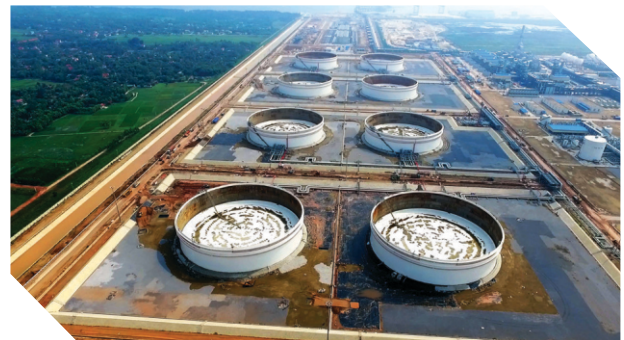
Nghi Son Refinery, Vietnam
