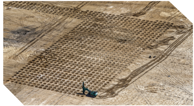
Jurong Island land preparation, Singapore
