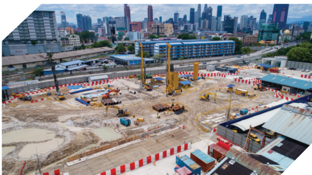
MRT Retaining System, Malaysia
