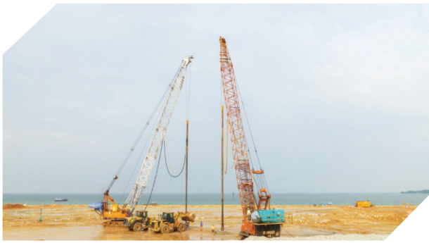
Karimun Petroleum Storage Terminal
