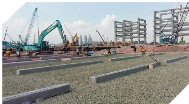
Petrochemical Complex, Malaysia
