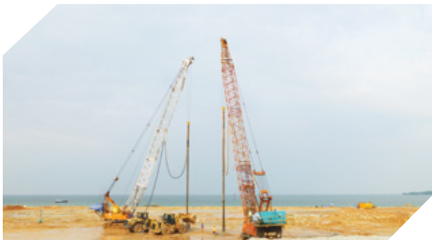
Karimun Petroleum Storage Terminal
