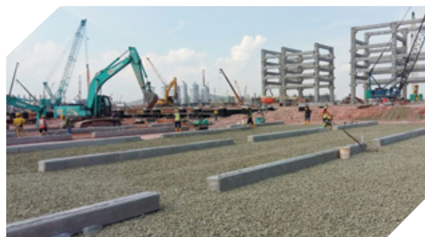
Petrochemical Complex, Malaysia
