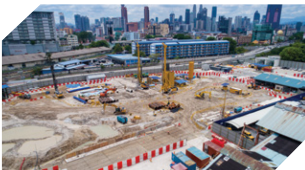
MRT Retaining System, Malaysia
