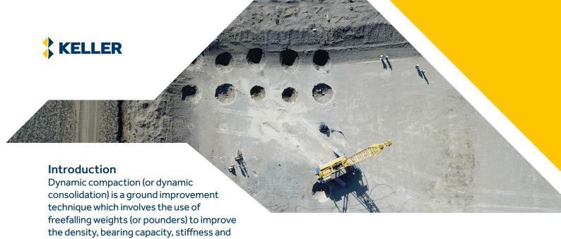
liquefaction resistance of granular soils. The choice of pounder and drop height depends on site conditions, compaction depths and materials to be compacted. Improvement depth of up to 12m can be achieved using dynamic compaction to provide allowable bearing pressures of up to 300kPa and settlements of 10-20mm for conventional structures.
